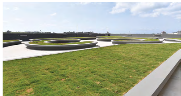
The green roof acts as an insulation layer to reduce solar heat gain into the building.
